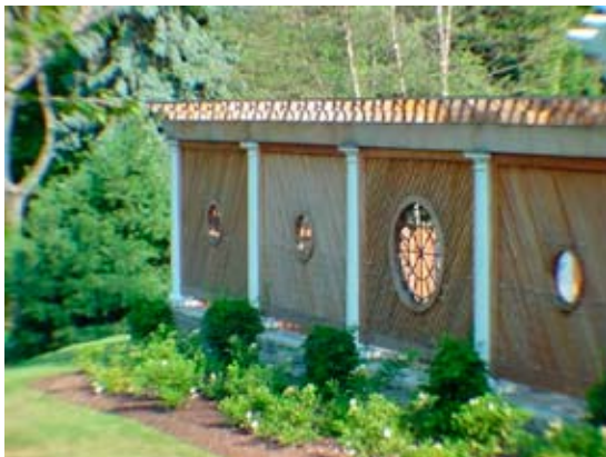
Lintel, Rafter & Purlin above Copper flashed Capital
