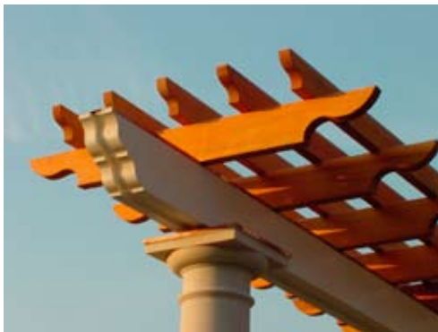
Colonnade with Tuscan columns, Cedar rafters & purlins
